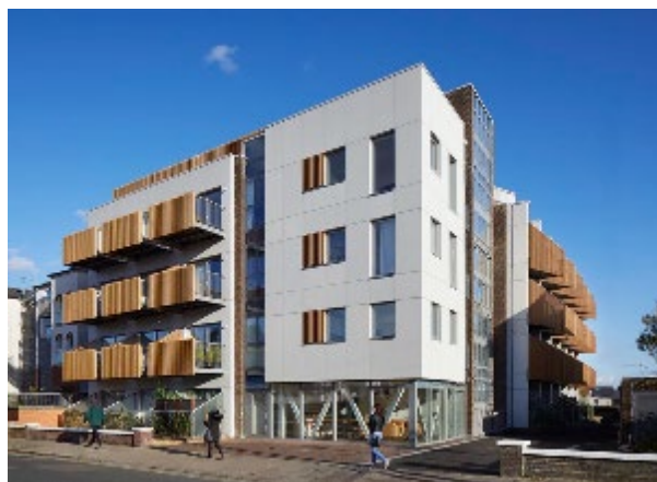
Below right: Paxton House in London. Former offices converted into flats. External circulation added to outside of building allows for greater number of apartments to be accommodated, each with a south or south west facing living space and balcony. Angled balustrade ensures privacy and maximises views from the interior. Walkways with chipped rubber ensures total acoustic dampening and acetylated timber longevity of building cladding. Croydon Council application 14/03324/P.
