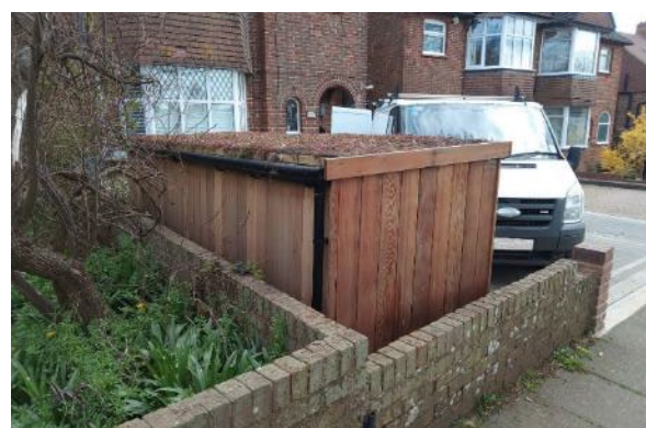
Above: Biosolar roof at The Ark, Noah's Ark Children's Hospice in London (left). London Borough of Barnet application 16/5151 . Green roof over bike shed in Hove provides habitat for wildlife, helps to insulate and make buildings more aesthetically attractive.
