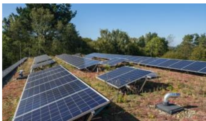
Above: Biosolar roof at The Ark, Noah's Ark Children's Hospice in London (left). London Borough of Barnet application 16/5151 . Green roof over bike shed in Hove provides habitat for wildlife, helps to insulate and make buildings more aesthetically attractive.
