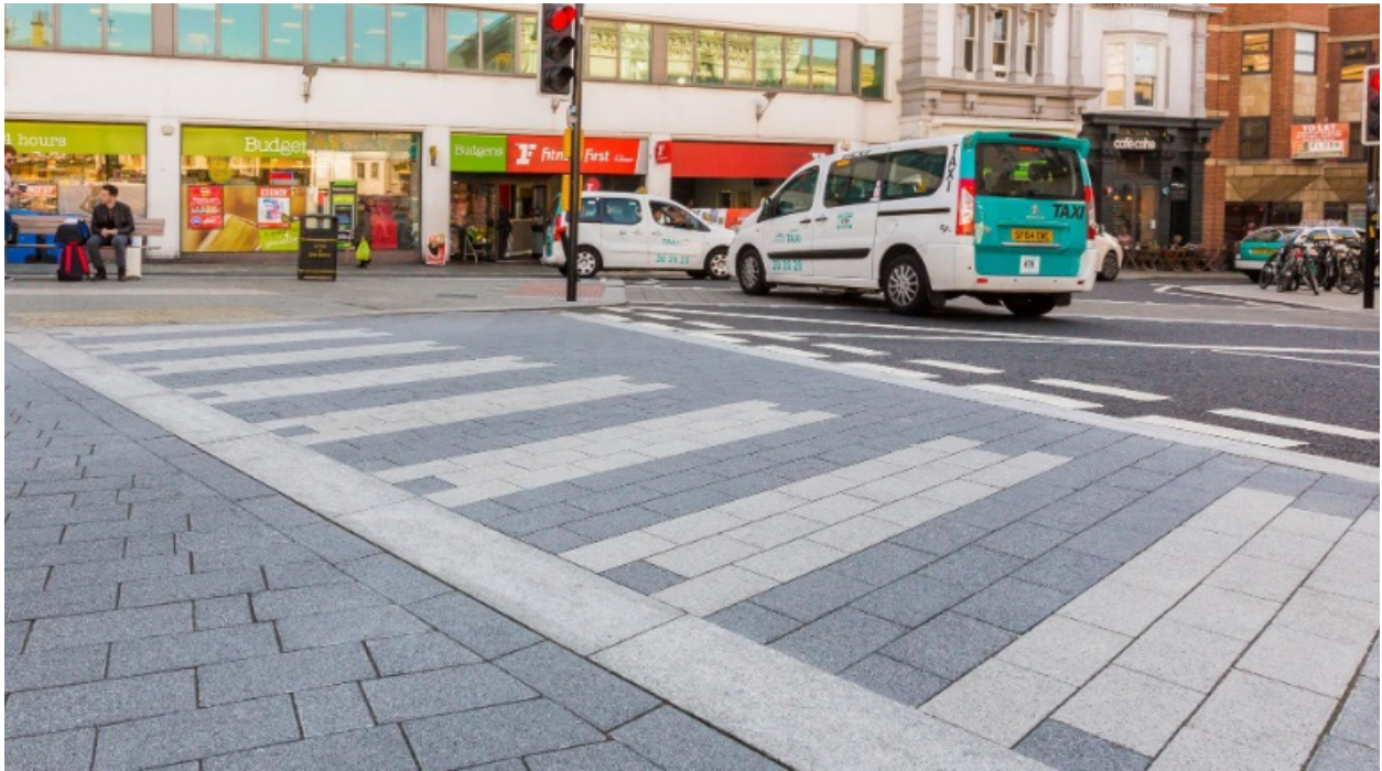
Above: Wide granite kerbs used to define edges of pedestrian realm and the carriageway and withstand level of intensity of pedestrian or heavy vehicle movements and resist damage and misuse. Brighton Station bus interchange, Brighton.
